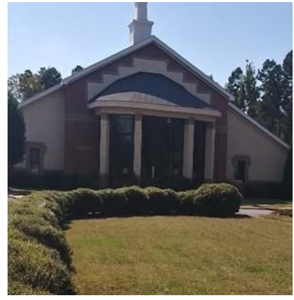
600 Capps Hill Mine Road The re-established institutional home
